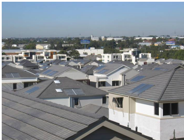
Figure 1 The Newington Roofline Photo courtesy BP Solar
