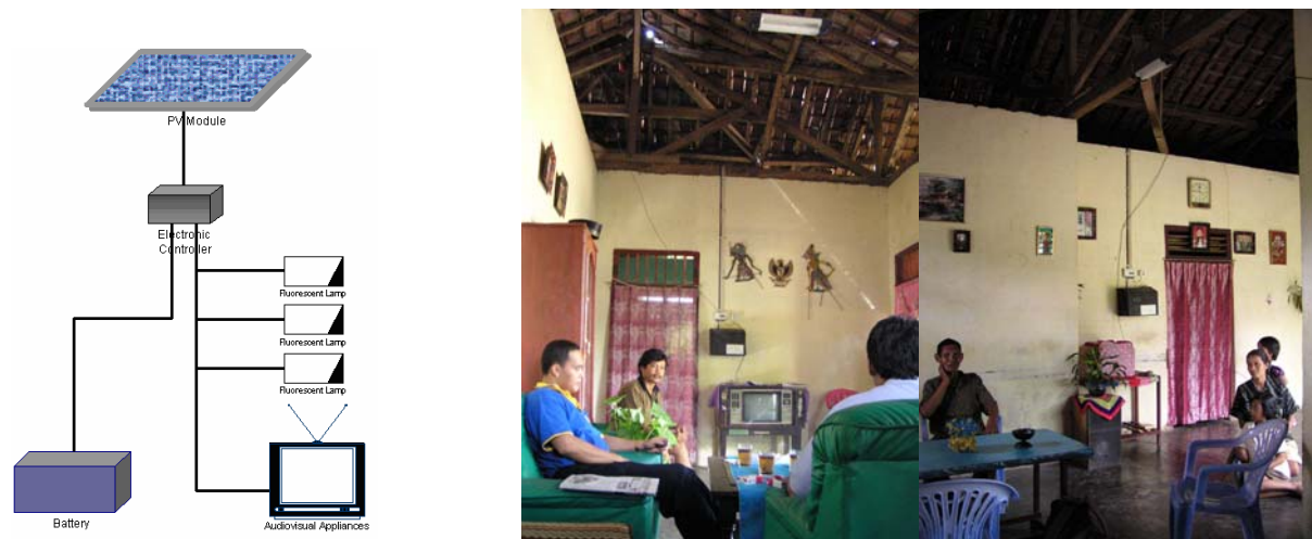
Figure 4a (left). A common PV lighting system package. Figure 4b (middle and right) PV lighting system installations in Lampung, Sumatra: The battery and the charge controller are located in the living room allowing practical observation of the charge state and the acid level of the battery by family members.
