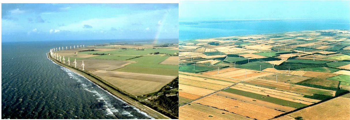
Figure 9. Contrasting wind farm layouts with respect to the effectiveness of smoothing of wind farm power output ( www.windpower.org )
