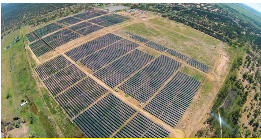
Barcladine solar farm. Credit: CATCON, Civil & Allied Technical Construction Pty Ltd
