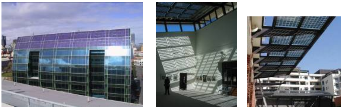
Figure 6,7 & 8: Melbourne University PV glass façade (STI, 2002), Kogarah Town Square translucent PV exhibition space and external PV awnings in Sydney (Kogarah Council, 2005).
