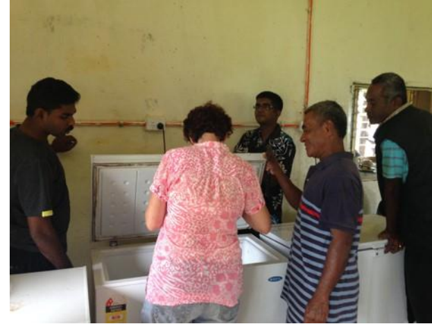
Solar PV powered Refrigeration Systems
