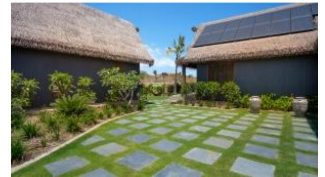
Six Senses Resort : Fully Solar + Tesla batteries
